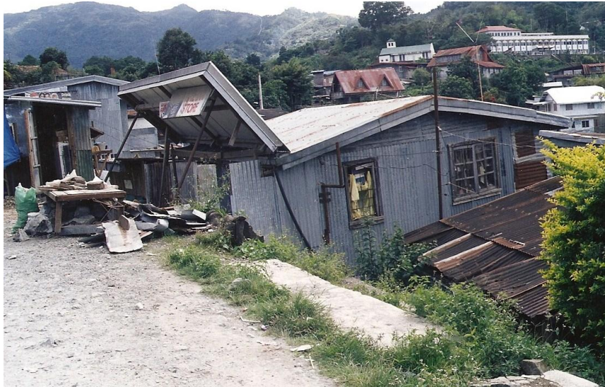
PHOTO 2: LIKE MANY, THIS HOUSE HAS SUBSIDED BELOW THE ROAD LEVEL AND IS UNINHABITABLE.
