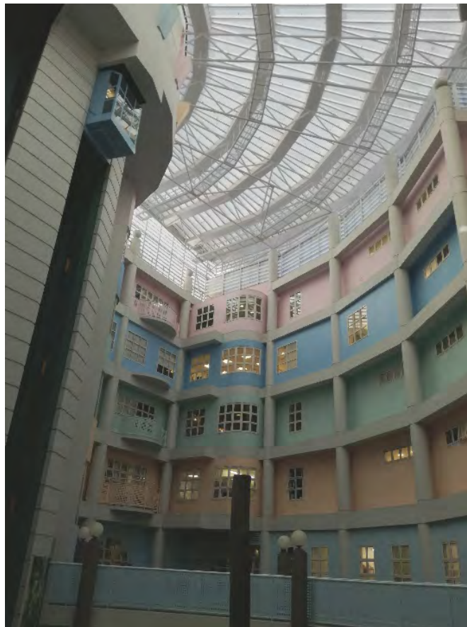
Figure 2. Existing Atrium interior walls
