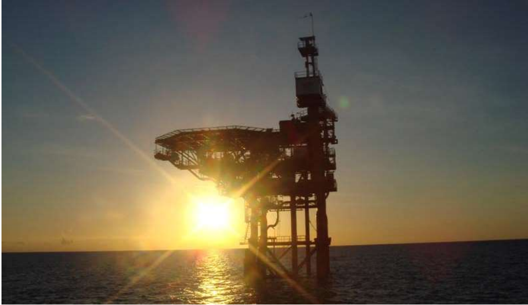
Figure 7.1: The Blacktip gas well platform, in the Timor Sea. Source: Monsta Cranes (2012).
