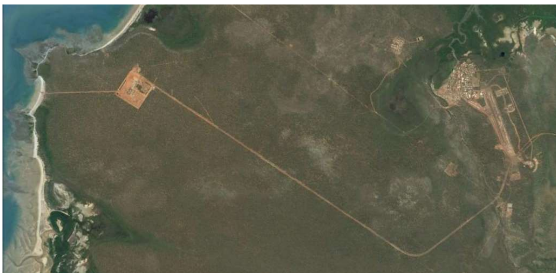
Figure 7.7: Blacktip's Yelcherr gas processing plant (on left) and the town of Wadeye (on right). Source: Google Earth (2016). Image reproduced under fair use of copyright.
