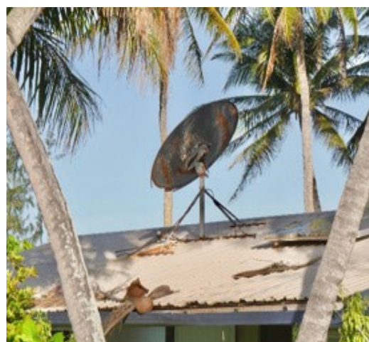
Figure 9: The proximity to salt water in Erub causes rapid corrosion of communications infrastructure
