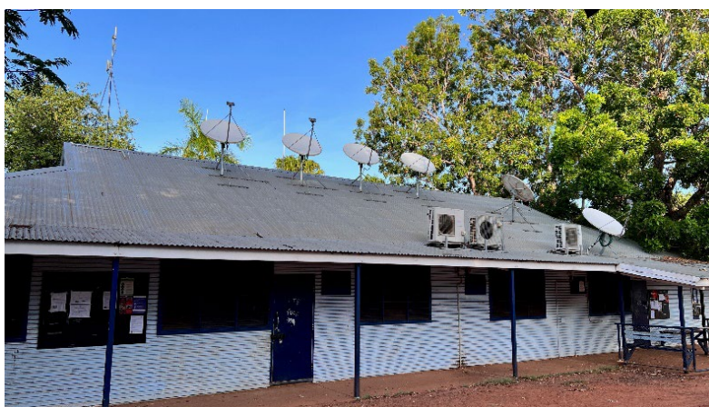
Figure 7: Four Sky Muster satellite dishes on the community office provide backhaul for the Wi-Fi mesh network.
