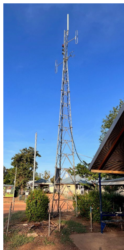
Figure 10: Radio broadcast tower adjacent to community office.
