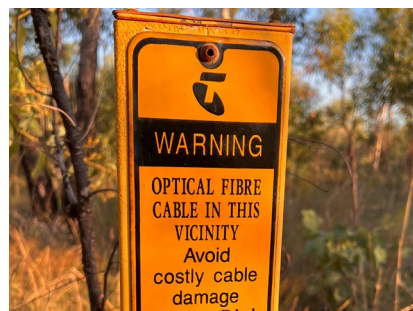
Figures 17 and 18: Julian using the public phone near the DAC community office; Yellow markers indicate the location of the fibre optic cable running alongside the Cape Leveque Road.
