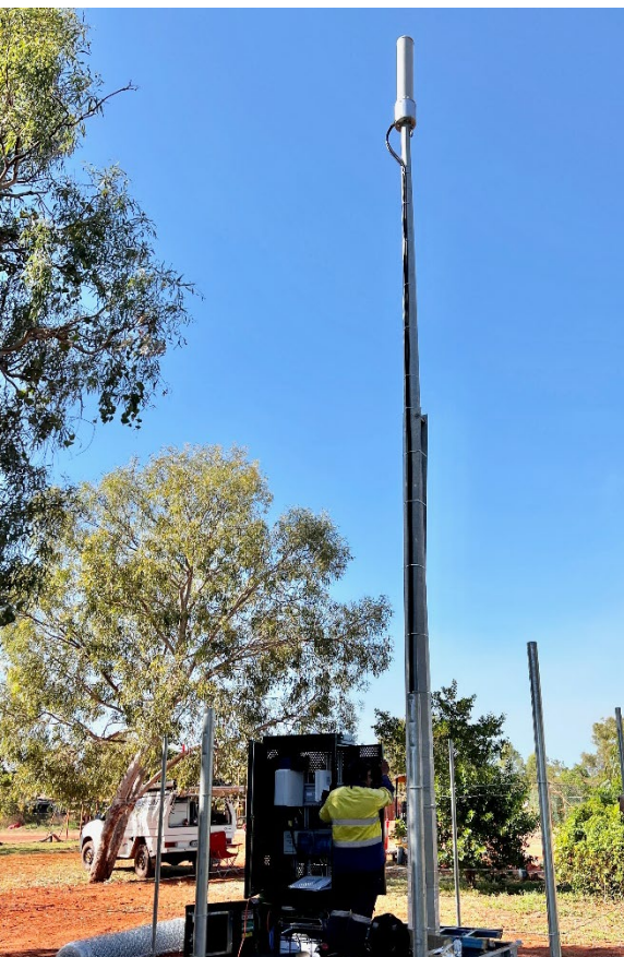
Figure 4: (left) A new 4G 700MHz small cell tower was installed near the Djarindjin community office in June 2022
