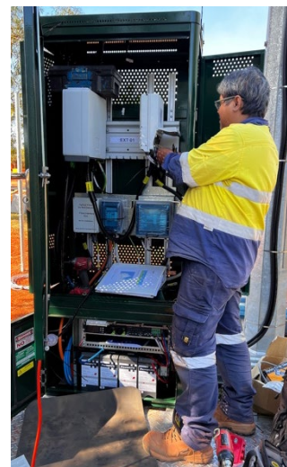
Figure 3: (right) Technician installing the mobile tower.
