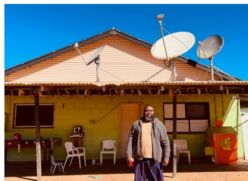
Figure 14: Mel Langdon at his home with Sky Muster (white) and VAST satellite (grey) dishes on the roof
