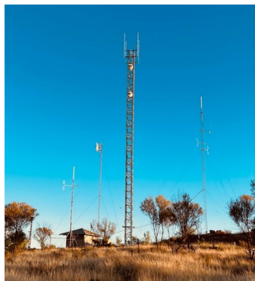
Figure 12: The new 40m 4G tower in Yuelamu, awaiting backhaul connection. The other towers are for HCRC microwave links (left of mobile tower) and radio broadcasting (right).
