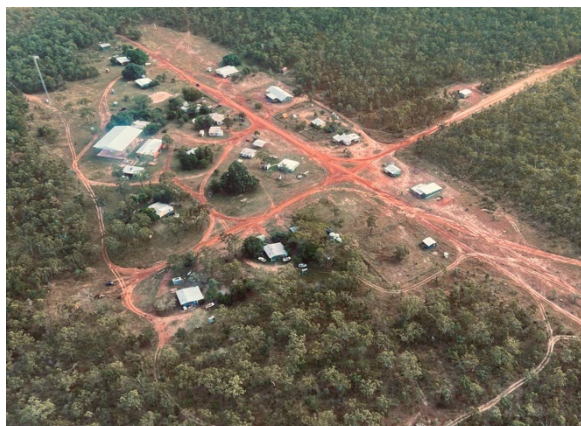
Figure 1: Aerial photo of Gängaṅ community
