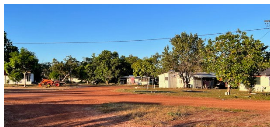
Figure 19: Only four of the 13 houses in Gängan still have a VAST satellite dish on the roof following housing upgrades
