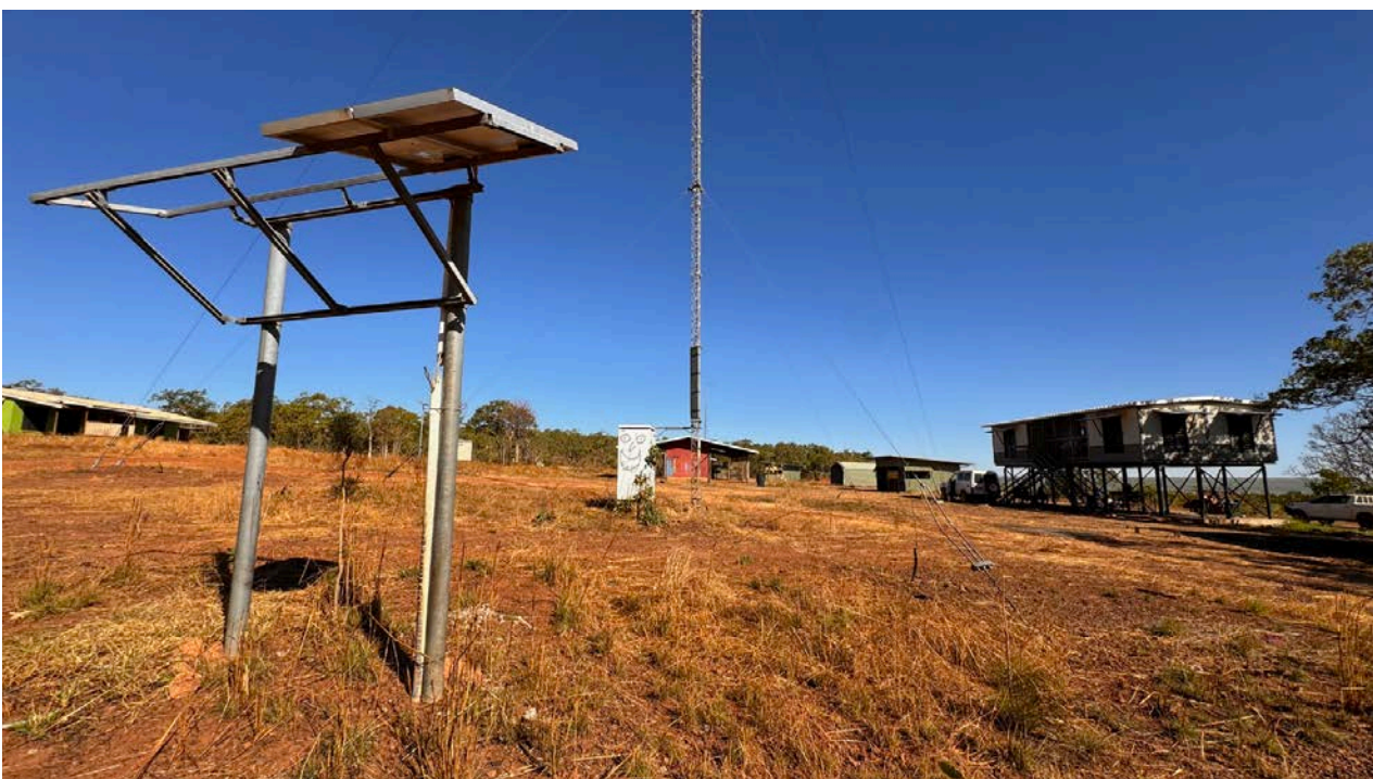
Old communications systems at Fossil Head homeland near Wadeye; microwave tower for Telstra phone and HF radio antenna. The more recent wall mounted phone hasn't worked for nearly a year.
