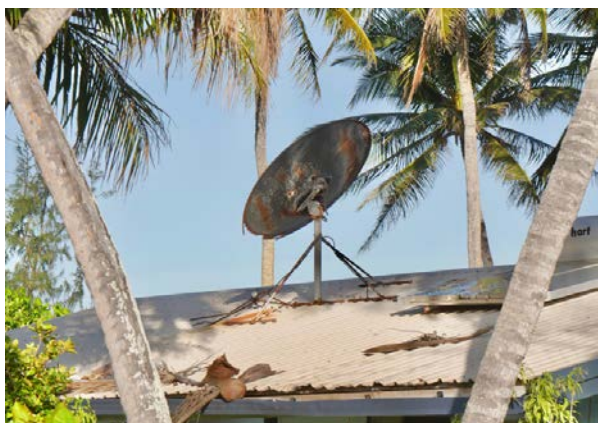
Rusted VAST satellite dish on house in Erub, Torres Strait
