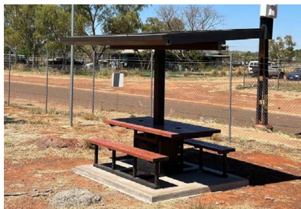
Newly installed solar Wi-Fi benches at Wuppa and Tingkarli CLAs, with wireless charging station (courtesy of Easyweb Digital)
