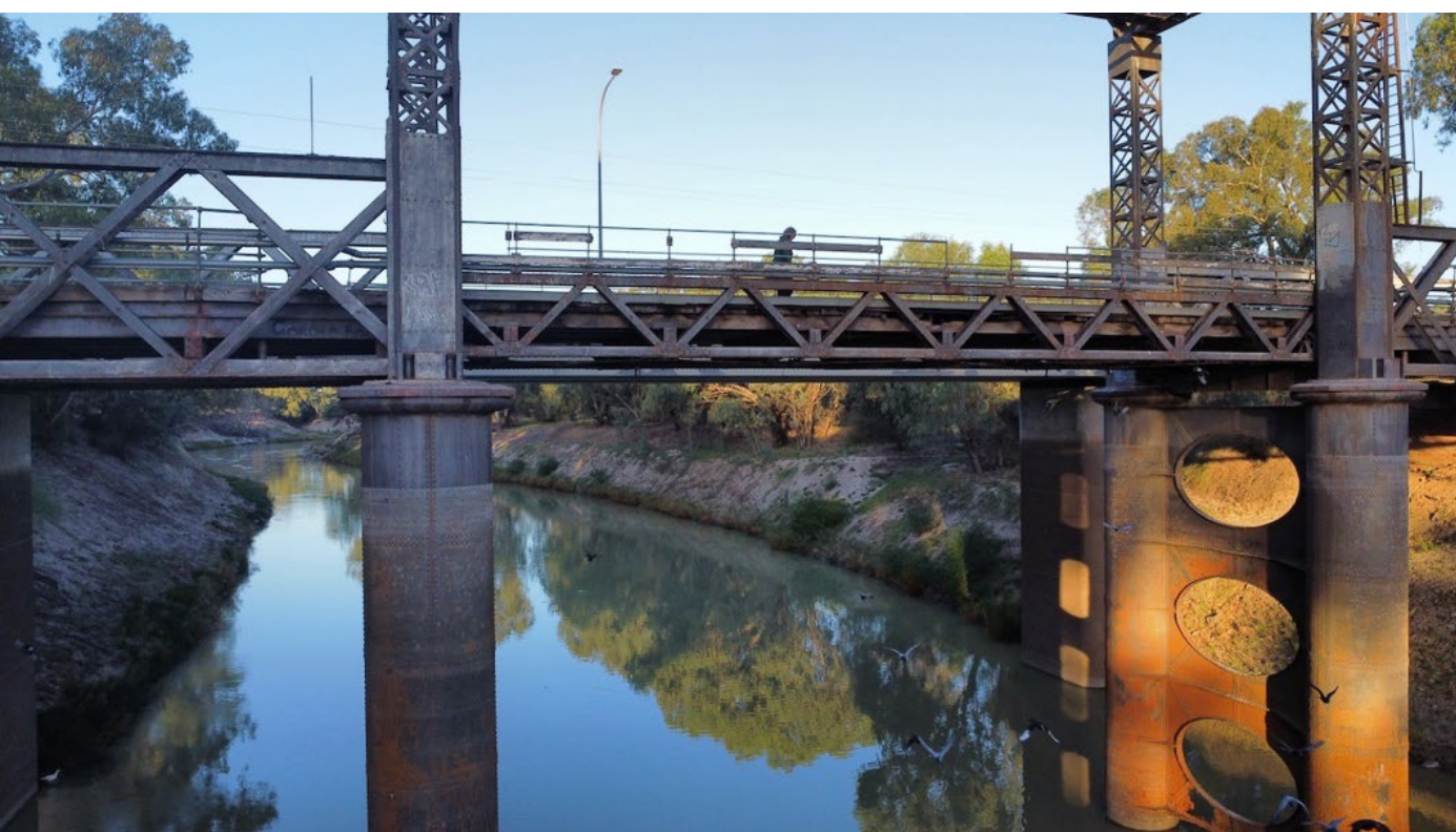
Figure 27: Bridge over Baaka (Darling River) on entry into Wilcannia
