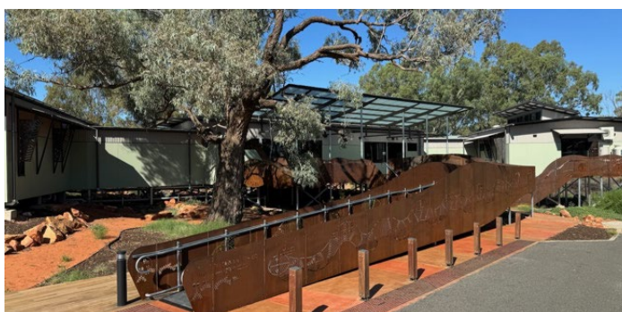
Figure 21: The New Maari Ma Health facility next door to Wilcannia Hospital, opened in 2023
