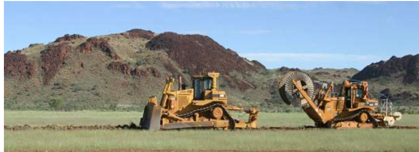
Figure 9: The fibre optic cable being laid near Blackstone community
