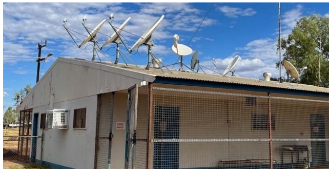
Figure 37: Three Sky Muster dishes on the Warakurna Community office provide backhaul for the Wi-Fi network
