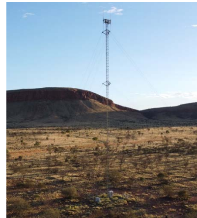
Figure 4: Warakurna mobile tower
