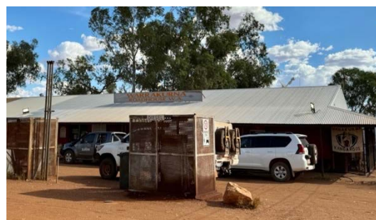
Figure 14: Warakurna Roadhouse is about 5km south of Warakurna community, opposite the multi-function police facility
